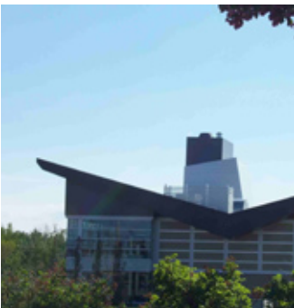
Strathcona County Centre in the Park community energy system power plant.
