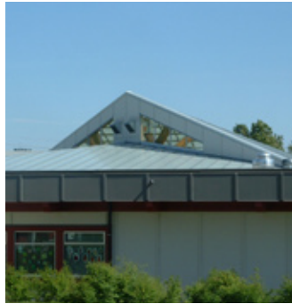
A clerestory window allows daylight to penetrate deep into the building.
