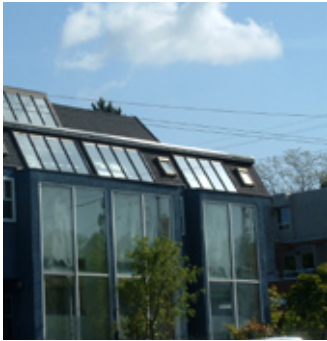
Buildings are oriented to capture the sun.
