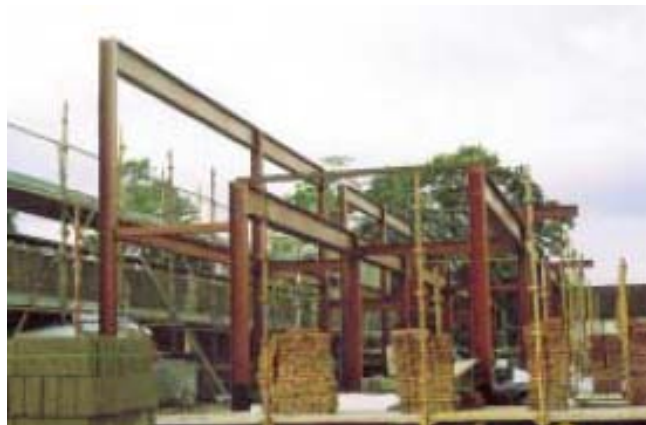
Reclaimed steel frame structure at BedZED - Credit BioRegional
