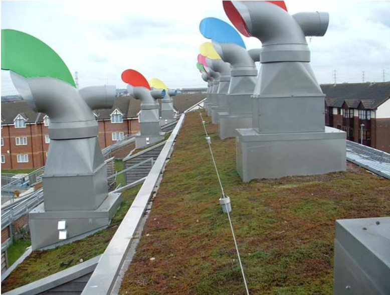
Zero maintenance sedum roofs at BedZED Credit BioRegional
