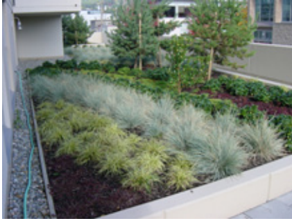
Fig. 16 The green roof on the Silva residential building in North Vancouver has a 27% reduction in the rate and quantity of stormwater runoff.
