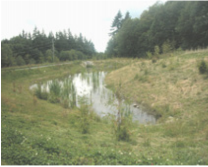
Fig. 13 A wet detention pond.
