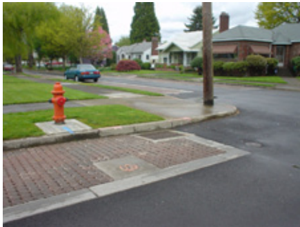
Fig. 17 Pervious pavement along streets in Portland, Oregon.
