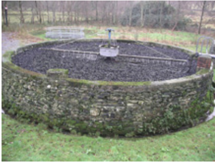
Fig. 10 Trickling filter sewage treatment bed.
