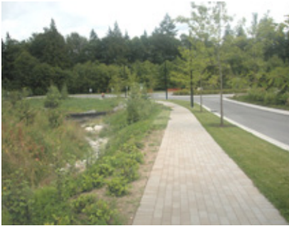
Fig. 14 An infiltration trench surrounding a high density residential development in Burnaby, B.C.
