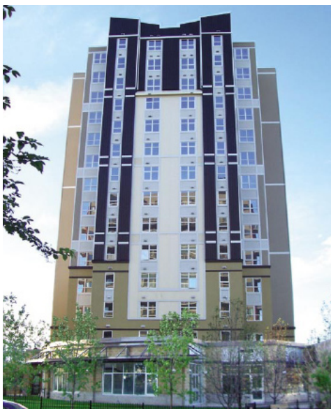
Figure 7: A SolarWall system installed at an apartment building in Calgary
