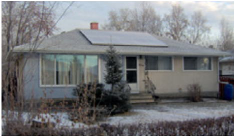
Figure 5: Strathearn House, a grid tied array, installed in November 2005, has been working well and in August 2006 the electricity bill for the house was $2.
