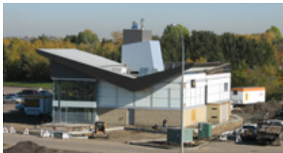
Figure 9: The City in the Park development within Sherwood Park includes a district energy system that serves the Strathcona County Hall, Festival Place, the Kinsmen Leisure Centre, and buildings constructed in Centre in the Park by Christenson Developments. Natural gas boilers are used to heat the water in the City in the Park district energy system.
