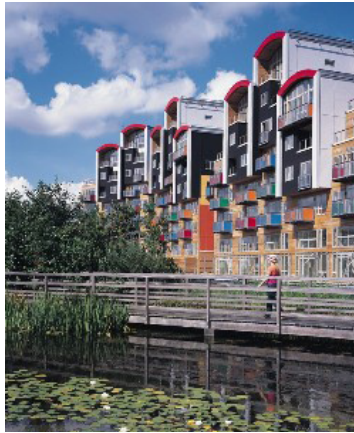
Figure 10: Greenwich Millennium Village uses a combined heat and power system to provide central heating, hot water and electricity to its occupants. It was the first UK private housing development to utilize CHP
