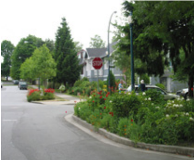
Fig. 7 Planted corner bulges in a residential neighbourhood.
