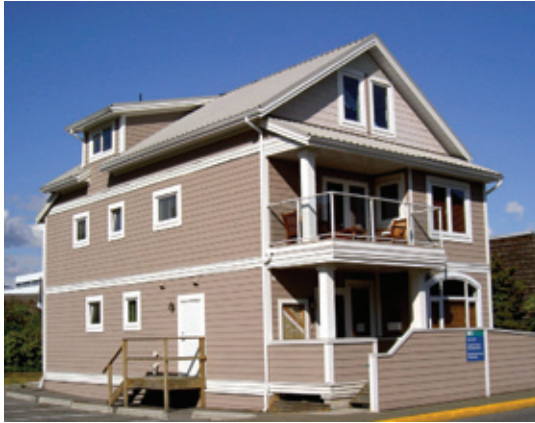
Figure 4: the Afresh home at BCIT Campus incorporates a flexible floorplan that can be adapted from a four-bedroom single family home to a two-bedroom duplex.
