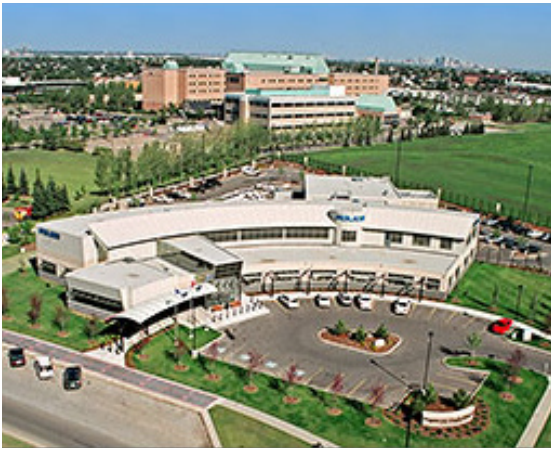
Figure 5: The new LEED Gold Edmonton Police Service South East Division Station diverted an impressive 99.67% of construction waste from the landfill.
