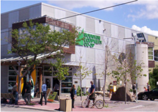
Figure 4. The Mountain Equipment Co-op in Ottawa reuses much of the original structure and was designed for deconstruction.
