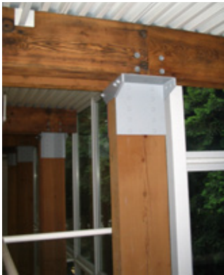
Figure 3. Slaved materials incorporated at the C.K. Choi Insitute for Asian Studies at UBC include 90-year old wooden beams, bricks, and stair railings.
